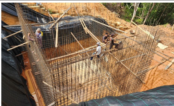
A large rain water tank being erected to provide drinking water for 8 houses.
