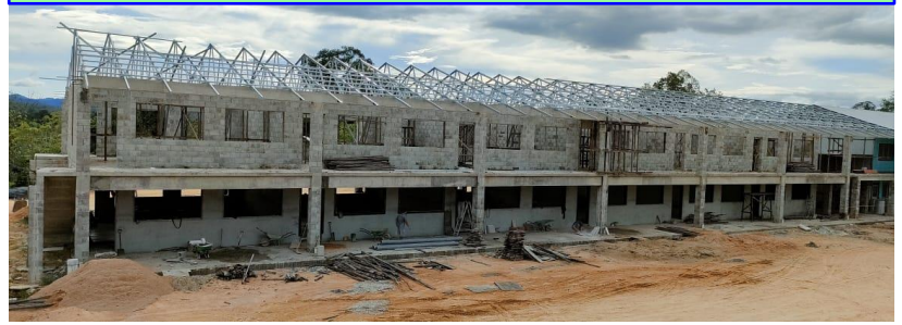
Above: The walls of the second floor of the new high school are being filled, all by hand. Below: Trusses are going up and roof sheets are being mounted as I am writing this. Hopefully we will have this building ready by July.
