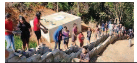
All helping with concreting one of the drains.
