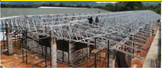
Two more children's homes almost ready for roof sheeting.
