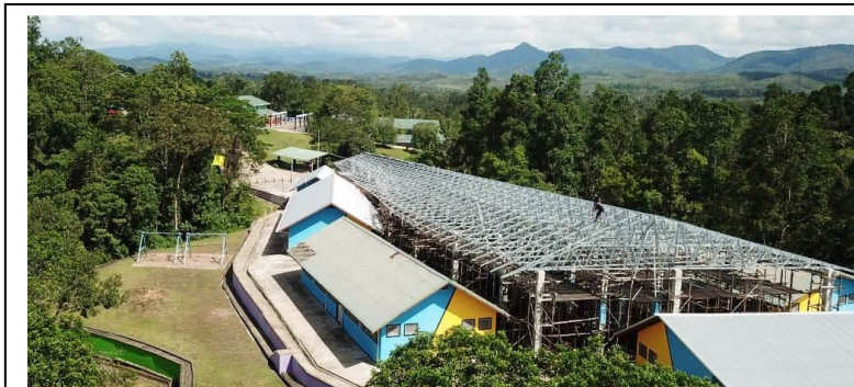
Trusses going up on our primary school undercover area.
