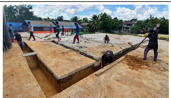
Building new foundations for our Abraham house.
