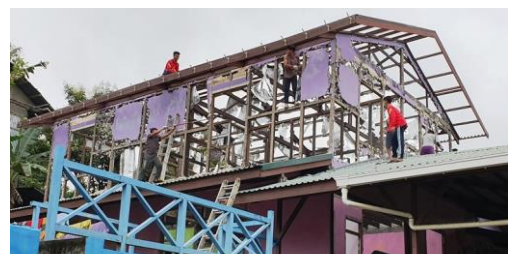
Demolishing our home in Nanga Pinoh.
